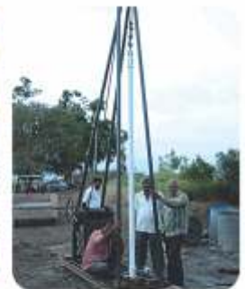
Lower the idol column pipes with chain pulley
