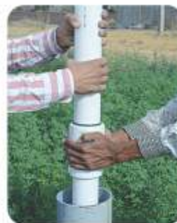
Hold coupler before loosening or tightening of pipes
